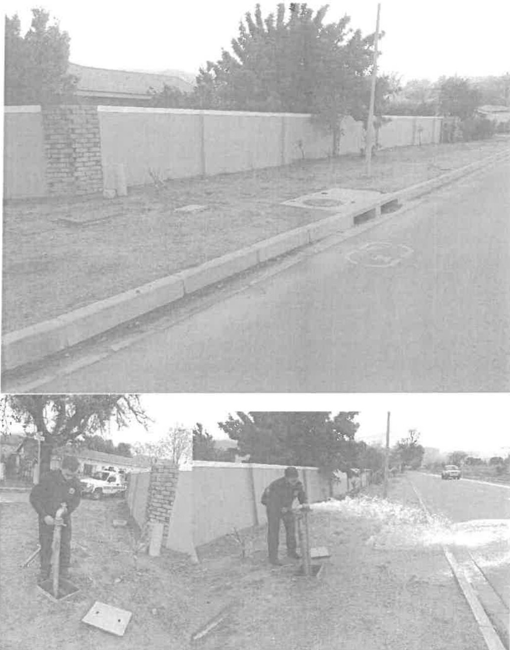
Figure 9: Hydrant marking and testing
