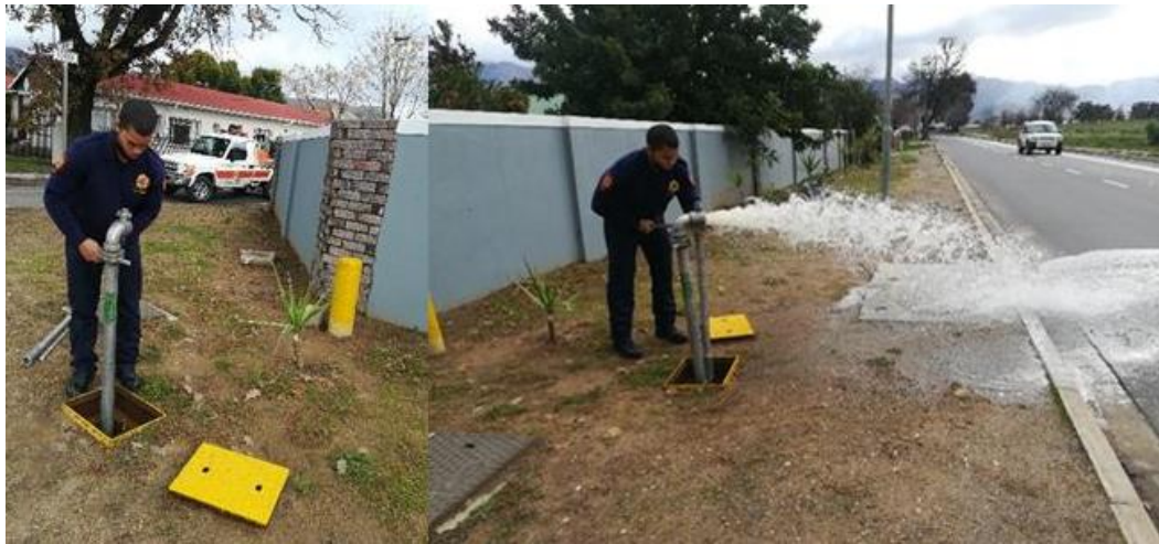
Hydrant Testing
